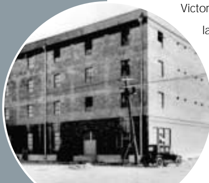
The 89-unit Victory Lofts development involves converting an existing warehouse that once stored Model T cars into 28 true loft units with 11-foot ceilings.
